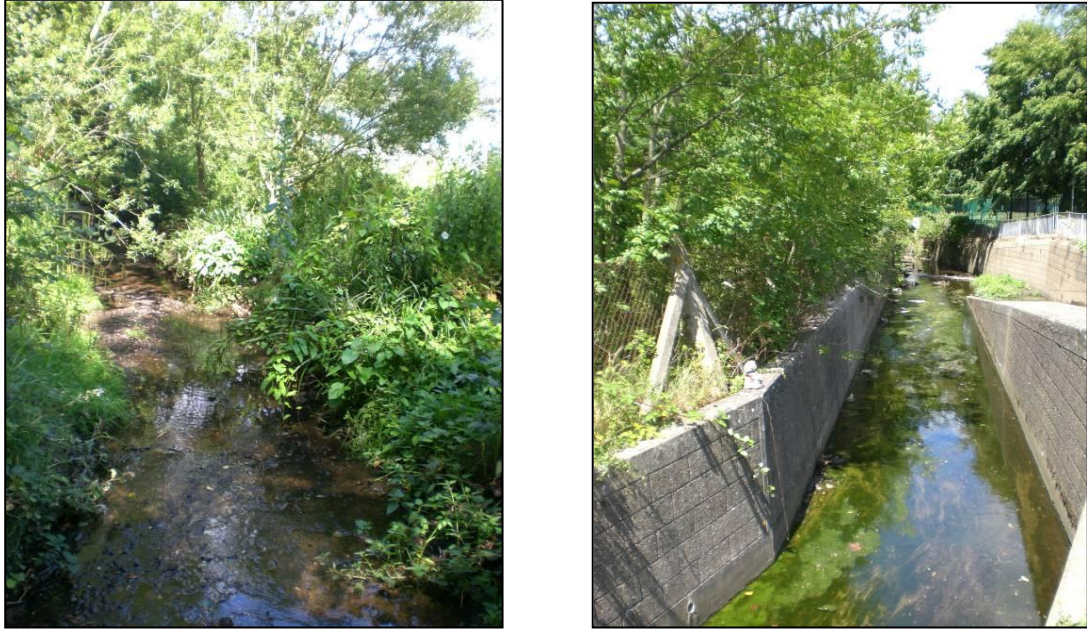
Figure 4.9: Photos of the restored (left) and unrestored (right) stretches of the River Quaggy at the Chinbrook Meadows site.
