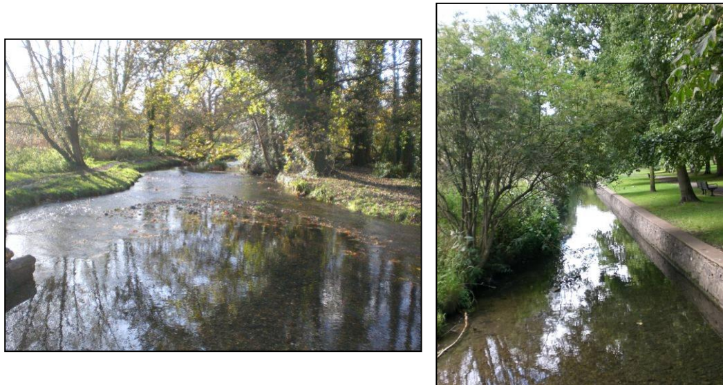
Figure 4.3: Photos of the restored (left) and unrestored (right) stretches of the River Wandle at the Beddington Park site.
