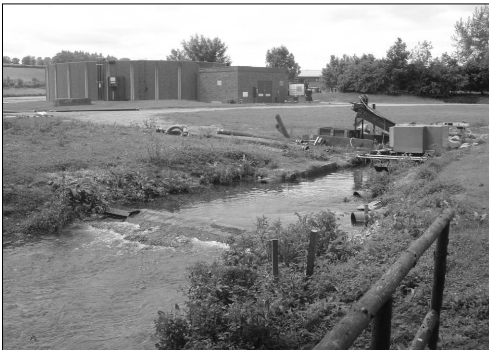
Plate 2.4. “Out” = “Outfall” heavily impacted site. Settlement tank in background.
