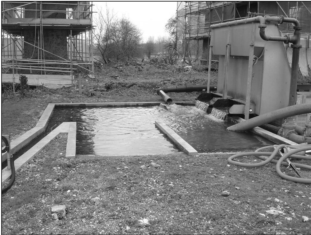
Plate 2.7. Sediment trap.
