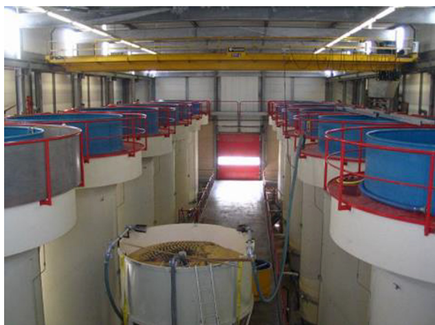
Fig. 1. Full-scale pellet softening reactors located at Waternet (Amsterdam, the Netherlands). The unit consists of 12 Amsterdam reactors with reactor diameter D = 3.0 m (van der Veen and Graveland, 1988).
