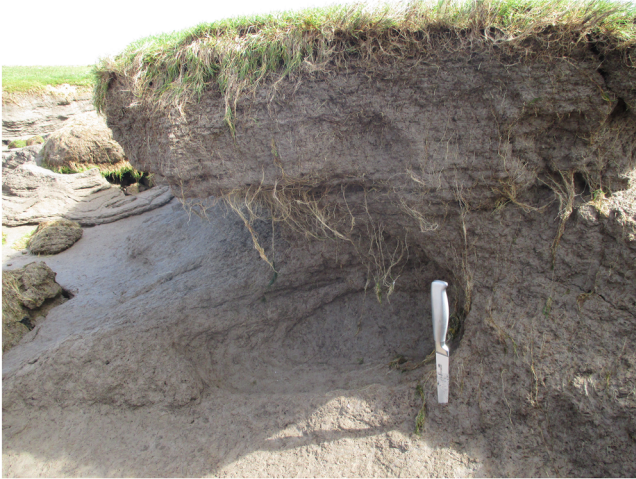
FIGURE 5. Example of undercutting at the base of the cliff, while the upper cliff overhangs and appears to be held in place due to tensile strength provided by the roots. Photo by I. Moeller taken at Warton Marsh, Morecambe Bay (UK) in July 2018. The knife in the photo is approximately 20 cm in length. [Colour figure can be viewed at wileyonlinelibrary.com ]
