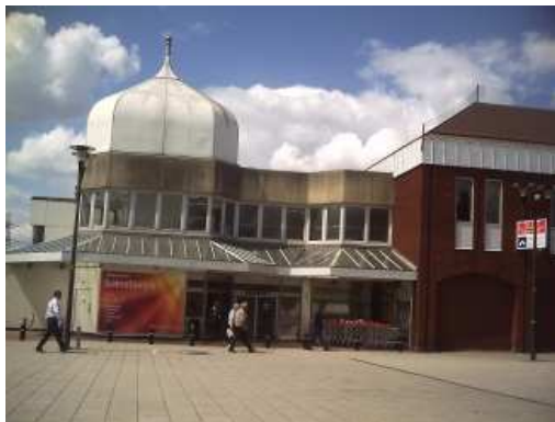
Plate 4.2: Photograph of Oldbury SavaCentre (by CT).
