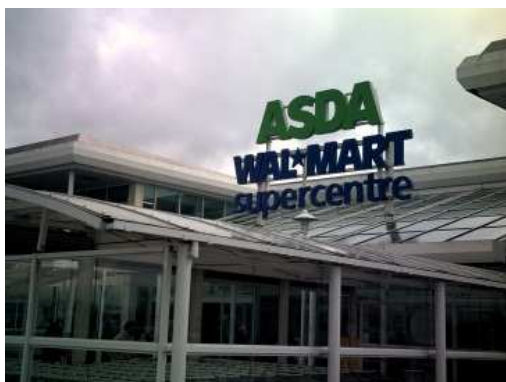
Plate 4.1: Photograph of Great Bridge Asda (by CT).
