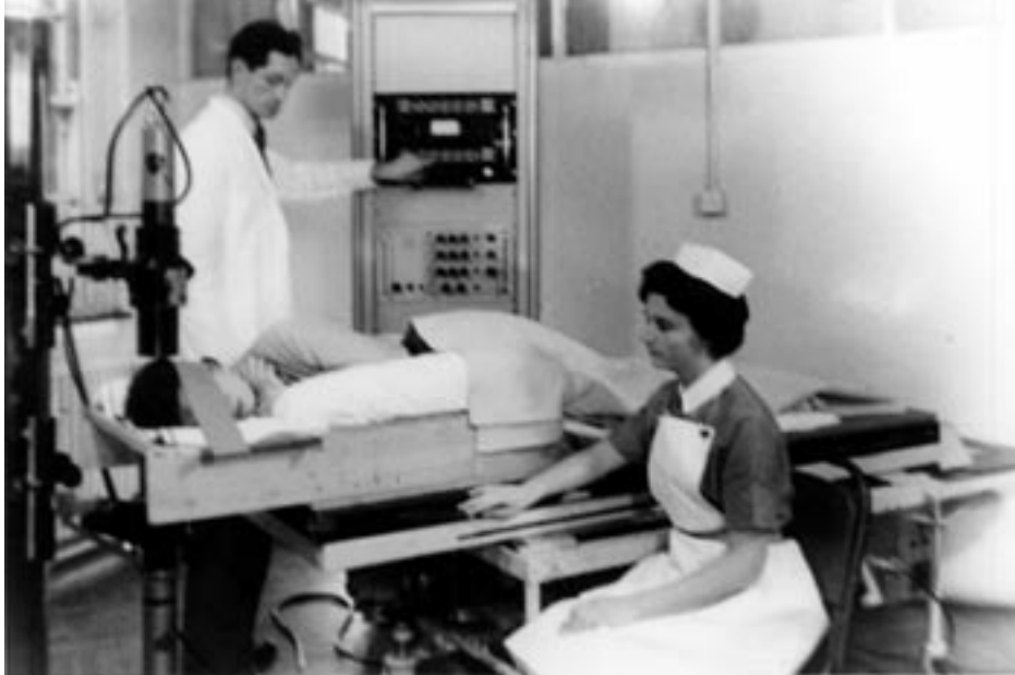
Figure 10: The first whole-body isotope scanner (homemade) in use for detecting a brain tumour, c. 1959. Mr Peachey is operating the electronics which has dekatrons display, at the Hammersmith Hospital, London. See notes 137, 138 and 139.
