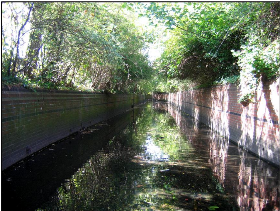
Figure 4.5: View of site 13 (WP west) immediately upstream of site 6, September 2009.
