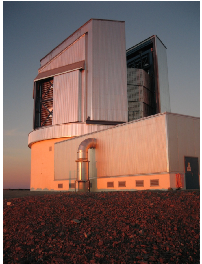
Fig. 14. VISTA enclosure seen from the southwest at sunset, with the auxiliary building in the foreground. Here the windscreen is fully raised, and an open ventilation door is seen on the left.
