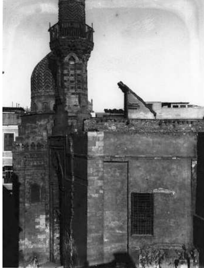
Figure 1.12: Bādahanj on the roof of emir Qānībāy al-Muḥammadī's Mosque (bl. 816/1314) in Cairo (© Creswell Archive, Ashmolean Museum, neg. EA.CA.1157)
