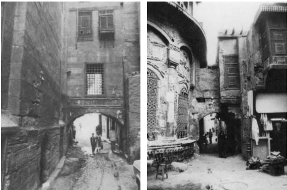
Figure 2.4: Ibn al-Rāmī's instructions to build a barrier wall to remove the auditory harm. Left: the situation before upon the complaint, right: after implementing Ibn al-Rāmī's solution (after B. Hakim 2008)
