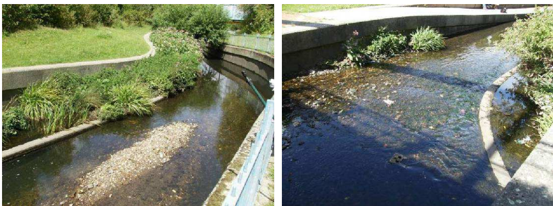
Figure 4.31 Views of the restored Pool river at Bell Green Gas Works (completed in 1994), showing indications of bio-physical recovery within the fully lined, enlarged concrete channel.
