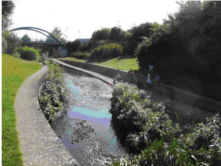
Figure 6.13 View of River Pool case study reach at Bell Green Gas Works
