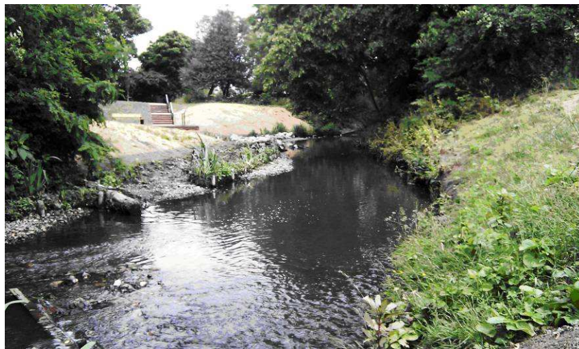
Figure 7.7 View of a section of the follow up restoration on the river Ravensbourne (Parklands project) in 2011 after success of the QUERCUS project completed in 2008.
