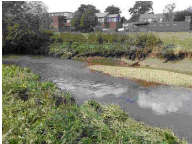
Figure 4.30 View of restored case study stretch on river Brent at Tockyngton Park: vertical eroding banks, mid-channel bar and riffle indicating morphological adjustments
