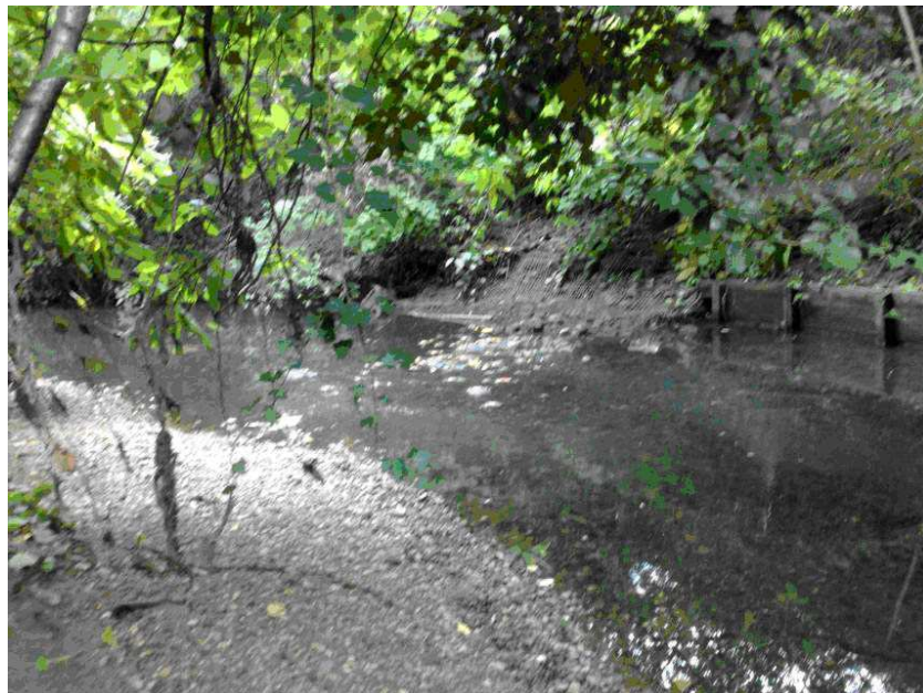
Figure 4.12 View of decaying toe board reinforcements with signs of physical recovery on the River Brent.
